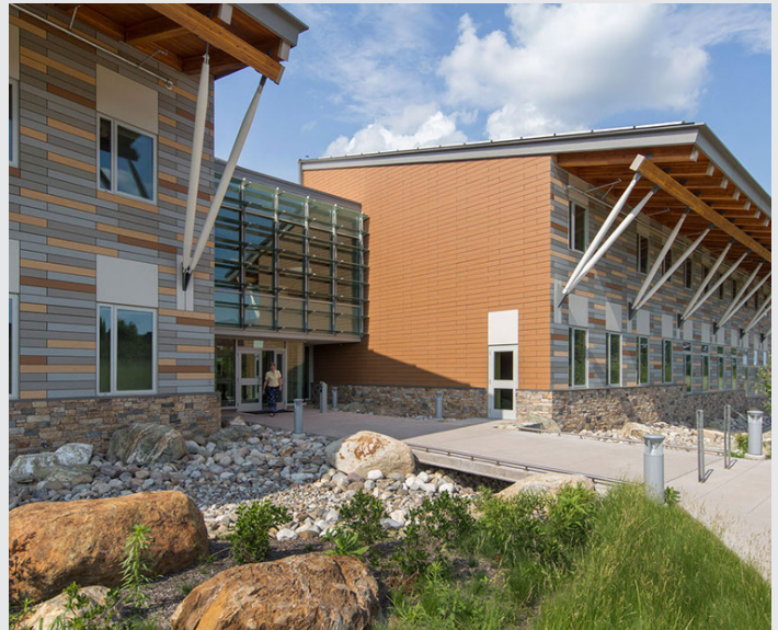
The Massachusetts Division of Fisheries & Wildlife Headquarters in Westborough, designed by Architerra, was one of the first netzero buildings in the state. The LEED Platinum certified building achieves zero net energy use by utilizing technologies that include photovoltaic panels and a geothermal system.
